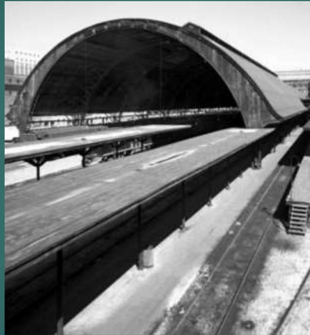
Large clear span structure that has to be designed so it can be removed to reach tracks
