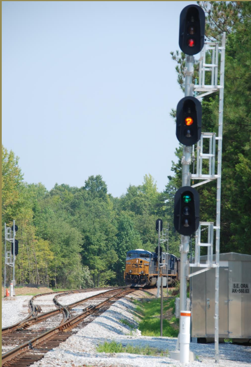
New CSX Color Lights South end Ora Note: Top two G/Y/R, bottom G/Lunar/R
