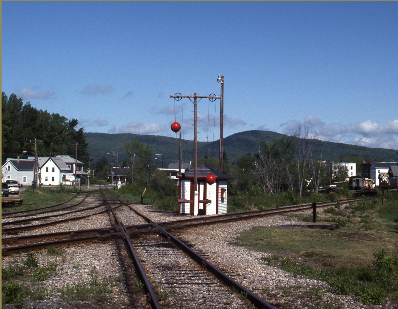
Ball Signal – Whitfield, VT Crossing of former B&M and MC lines Believe several lasted into 1950's
